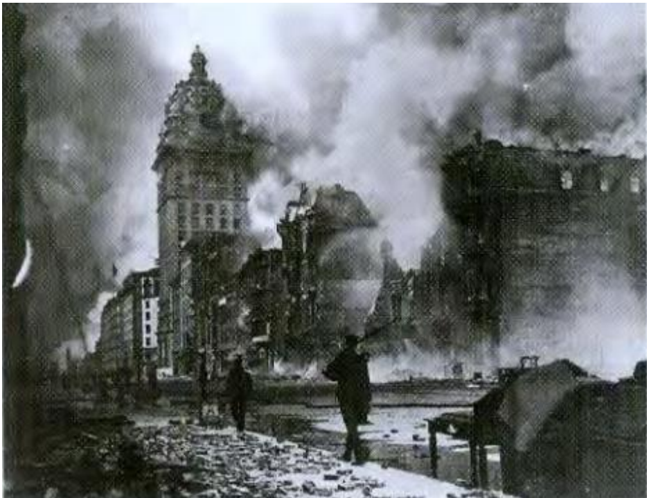
After the earthquake
